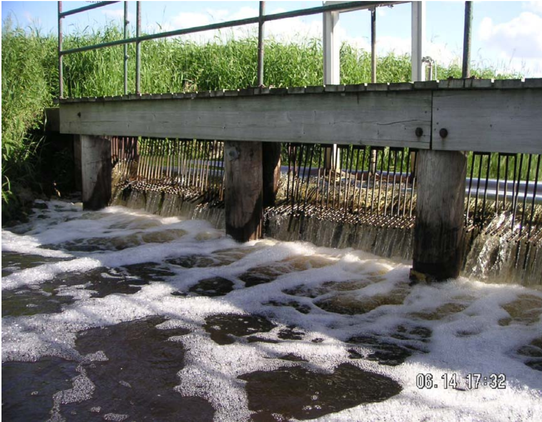
Figure 5. Highway 13 Wetland Fish Barrier (Prior Lake Spring Lake Watershed District, located in Scott County)
