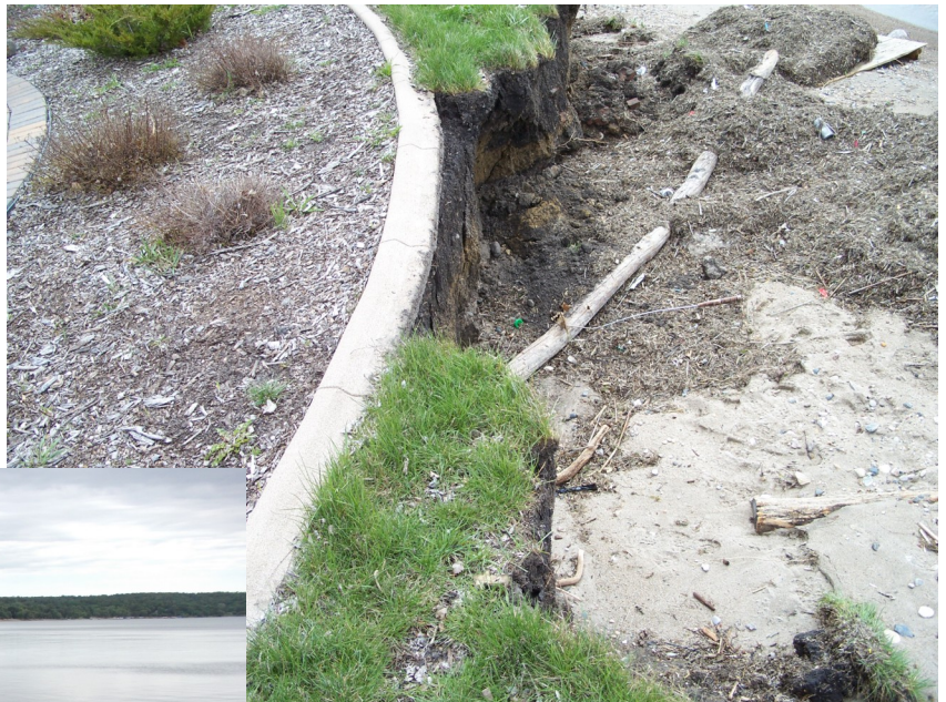
Example of Lake Minnewaska lakeshore erosion from high water, wave and wind action before and after.
